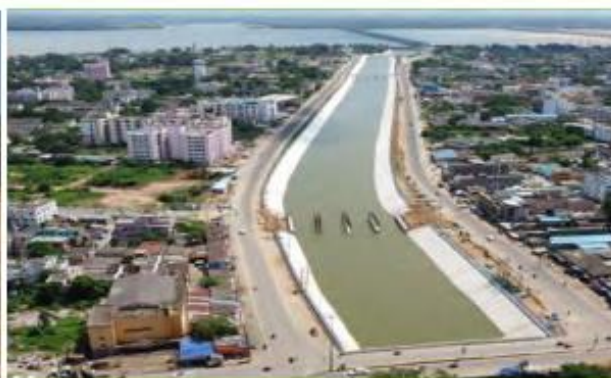
Taladanda Main Canal
