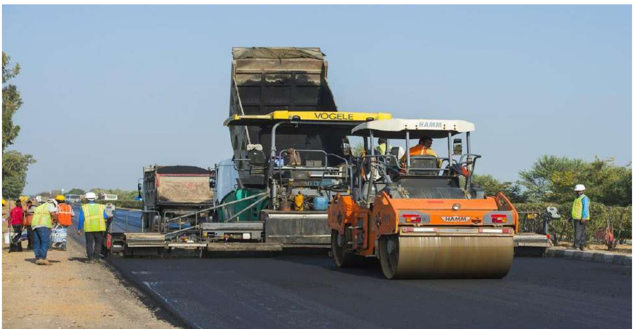
Figure 4. Major Maintenance & Repairs
