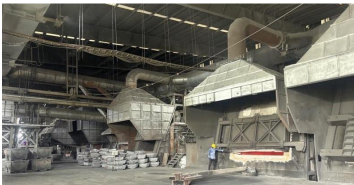
Exhibit 2: Liquid Metal Furnace & Storage
